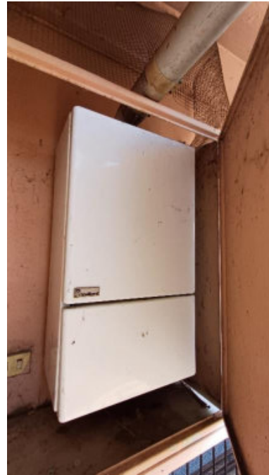
Caldaia a gas
